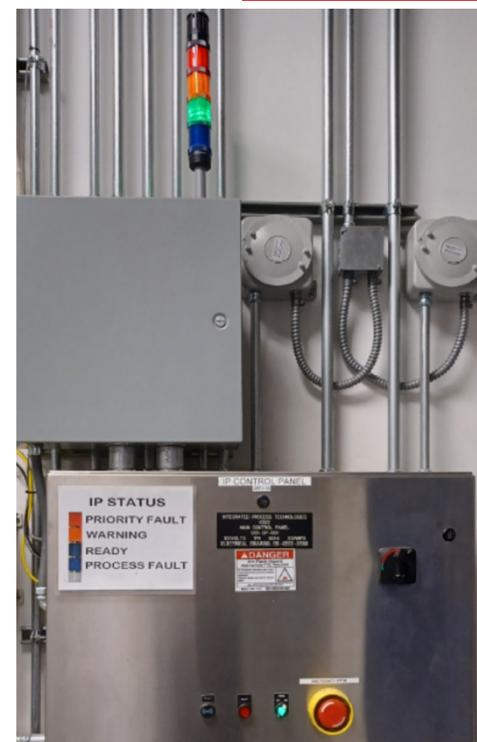
Automated process control with visual, audio and text message alarm capability
