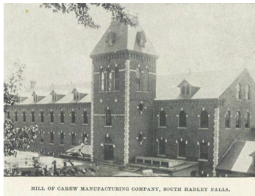
Carew Manufacturing Company, ca. 1874 at rebuilding.
