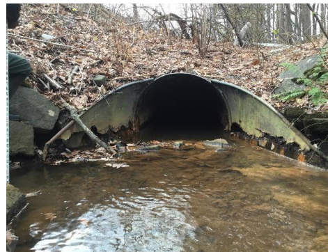
Image 2: Existing structure outlet during field visit on November 25, 2020. Note the gaps on either side of the culvert where erosion and piping may be occurring and the damage to the flared end section.
