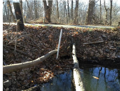
Image 1: Existing structure inlet during field visit on December 10, 2020, showing only the top of the pipe. The rest of the inlet is buried under sediment and debris.
