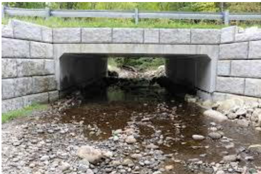
Image 3: Example of a box culvert (Maine Audubon).
