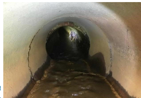
Image 2: Existing structure outlet during field visit on November 25, 2020. Note the gaps on either side of the culvert where erosion and piping may be occurring and the damage to the flared end section.
