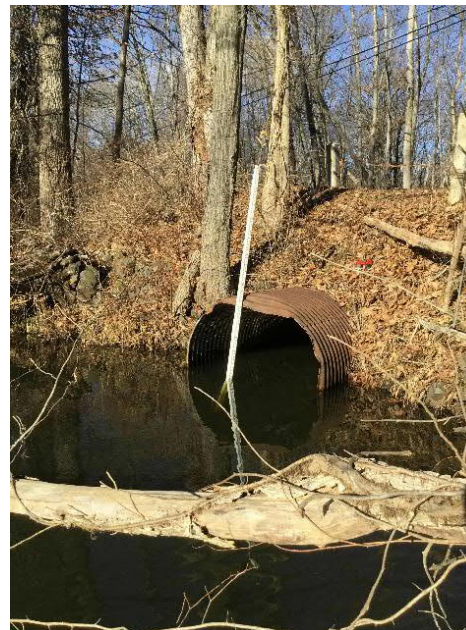
Image 2: Existing structure outlet during field visit on December 10, 2020.
