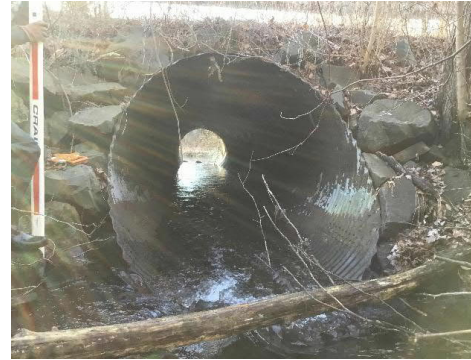
Image 1: Existing structure inlet during field visit on November 24, 2020.
