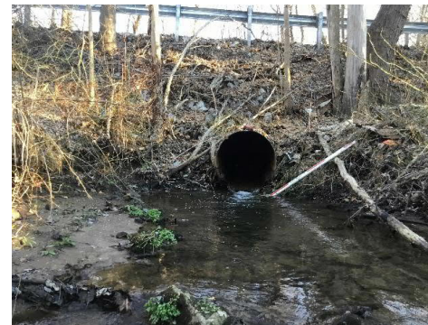
Image 2: Existing structure outlet during field visit on December 4, 2020. Note the large scour pool, eroded banks, and perched outlet.
