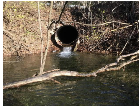
Image 2: Existing structure outlet during field visit on November 24, 2020. Note the large scour pool, eroded banks, and perched outlet. Also note the change from concrete at the inlet to corrugated metal at the outlet.
