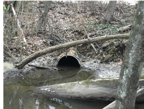
Image 2: Existing structure outlet during field visit on December 9, 2020. Note the severely eroded banks.
