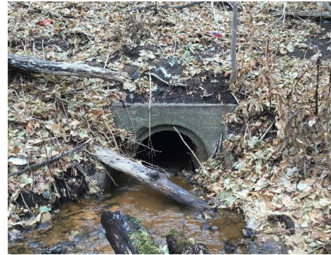
Image 1: Existing structure inlet during field visit on November 25, 2020, showing a blockage causing a drop into the inlet and erosion of the banks to either side.
