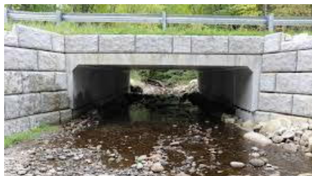
Image 3: Example of embedded box culvert (Maine Audubon).
