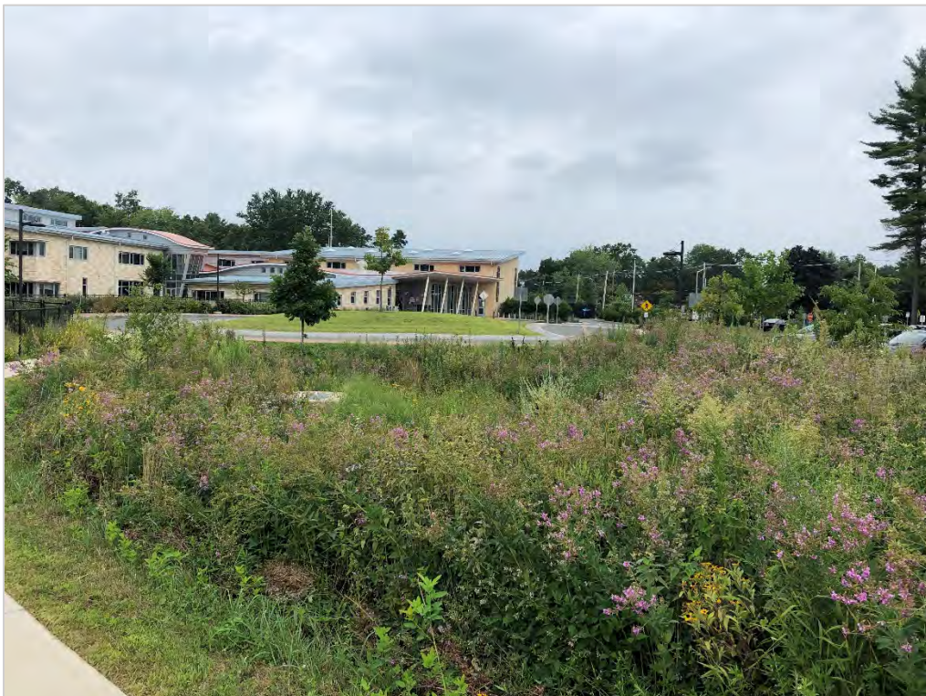
Bioretention area and pollinator garden serves as stormwater management system at Plains School parking lot
