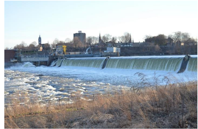
Holyoke Dam between South Hadley and Holyoke, MA
