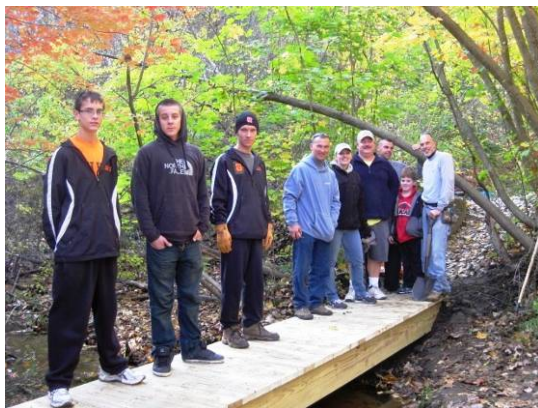
New Bridge and Work Crew at Black Stevens Conservation Area.
