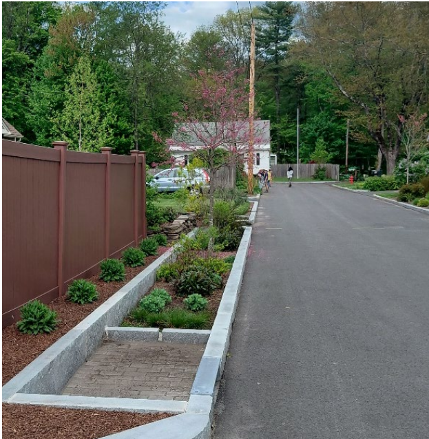
Streetscape rain garden in the right-of-way. A curb cut (foreground) channels street runoff into a forebay (brick-lined), where sediment settles before the water overflows into the planted area for infiltration. Photo source: Kate Cholakis.
