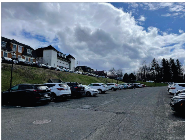
Image 3 View from Lower Parking Lot to Upper Parking Lot and Mixed-Use Buildings
