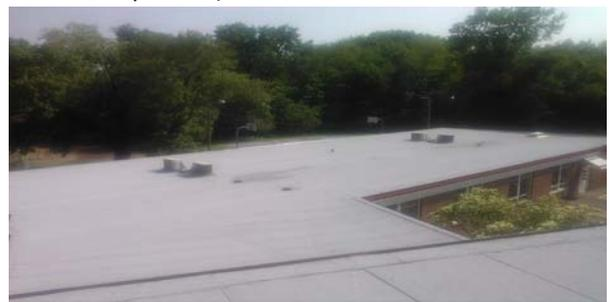
The membrane has a twenty year warrantee and we received failure instructions to contact Trimco as to any leaks. There is a few "punch list items we requested, including the installation of a scupper drain on the front side of the cupola stand to allow better drainage for standing water in that area.
