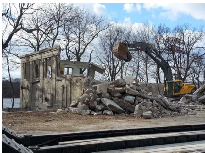
Filter Building Demolition – February 4, 2013
