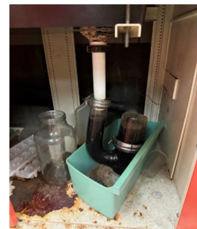
Neutralization Trap
