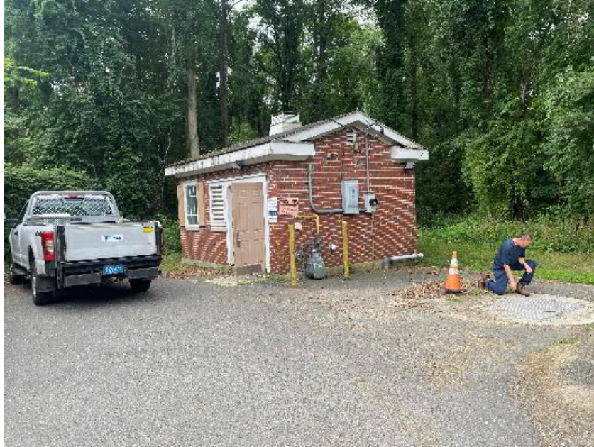
Stony Brook Pump Station: Pump House.
