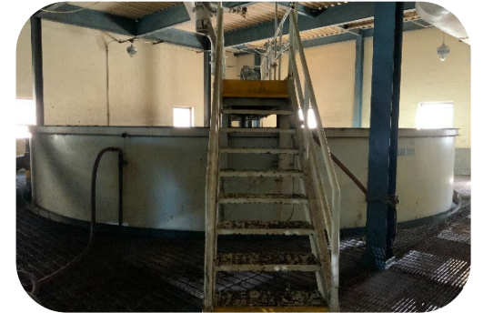
Gravity Thickeners
