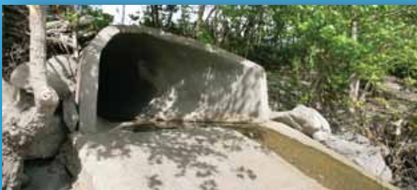
Storm Drain Outfall
